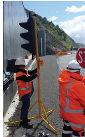
Slide lantern into the centre locking column with assembly facing away from traffic
