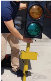
Use two hands to lift traffic lantern onto base
