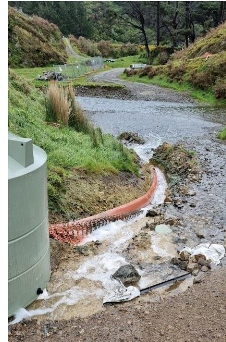
Overflow into stream
