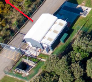
UV Treatment Building
