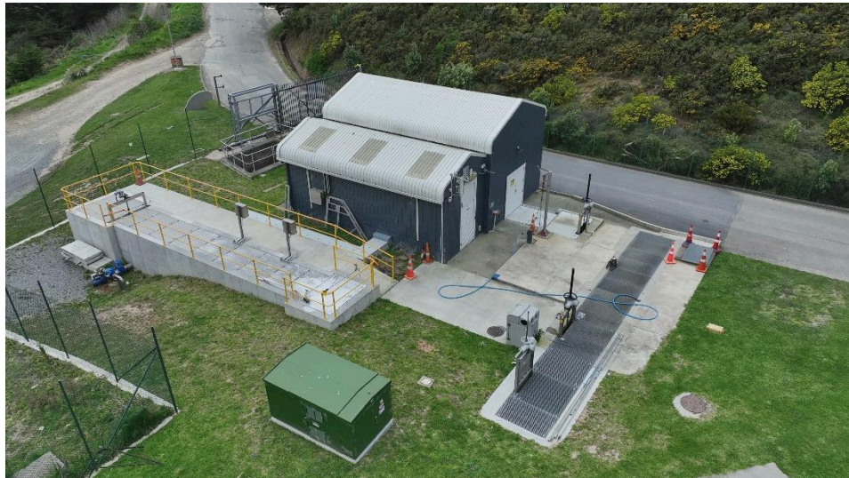
Figure 11: Ultraviolet System Building
