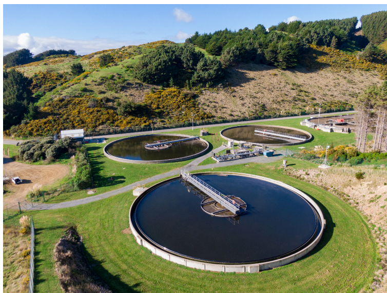
Figure 10: Secondary Clarifiers
