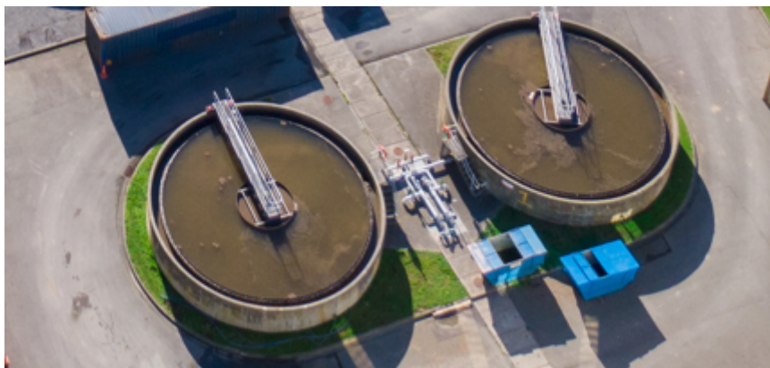
Figure 12: Sludge Thickeners
