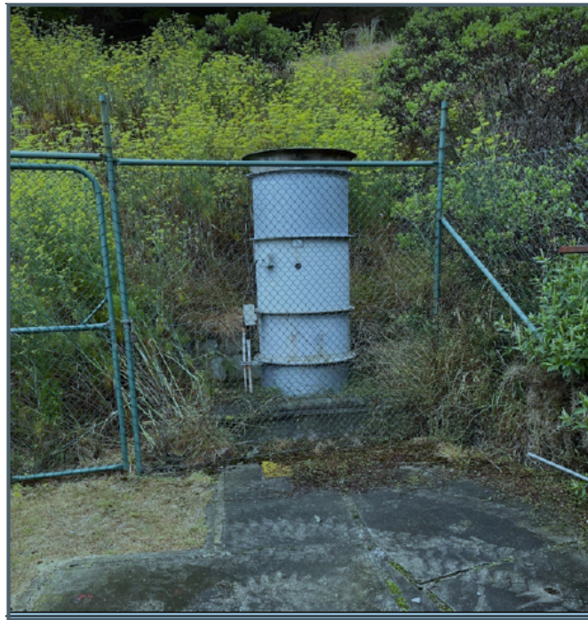
Figure 5. Tunnel Inlet Vent
