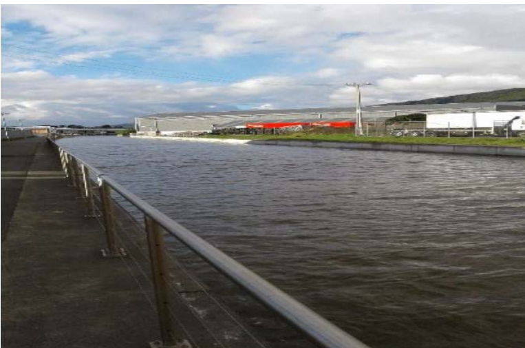
Figure E-8: Main plant overflow outlet on 17 July 2019
