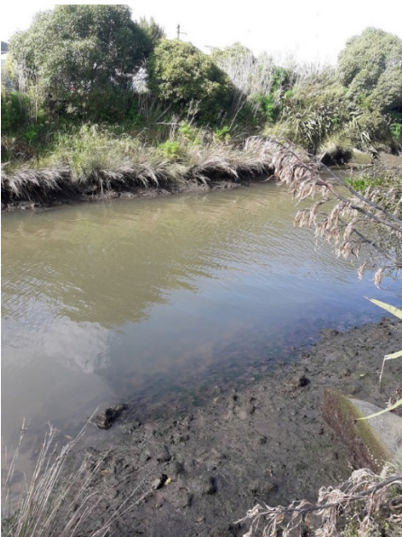
Figure E-31: Site C. Bell Road Bridge on 12 November 2019
