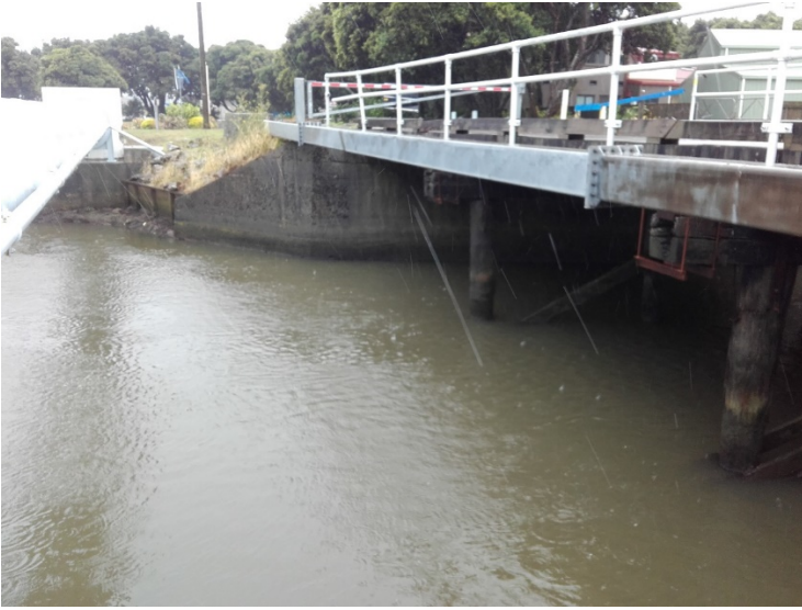
Figure E-50: Site C. Bell Road Bridge on 29 March 2020
