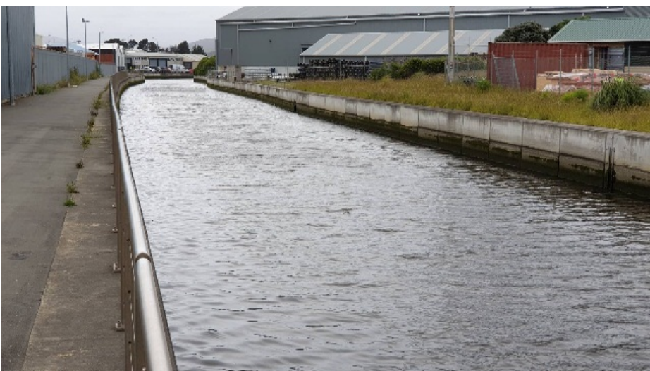
Figure E-40: Main plant overflow outlet on 18 December 2019
