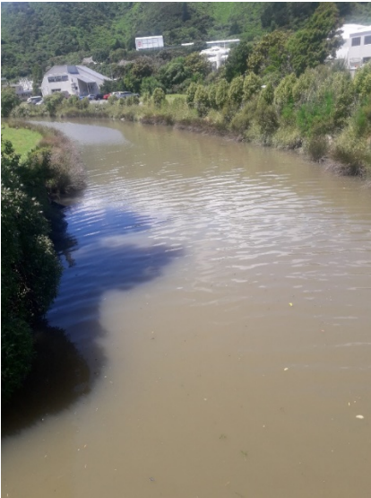
Figure E-39: Site C. Bell Road Bridge on 09 December 2019
