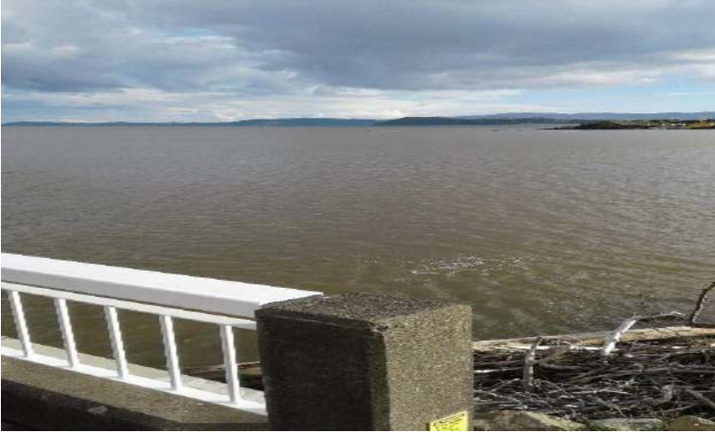
Figure E-9: Site A. Port Road on 17 July 2019
