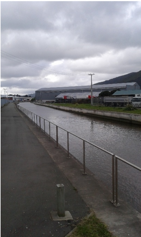
Figure E-17: Site A, Port Road on 14 August 2019
