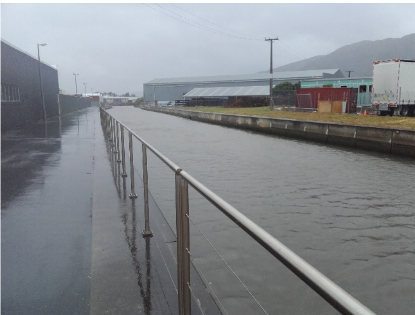
Figure E-43: Main plant overflow outlet on 28 March 2020
