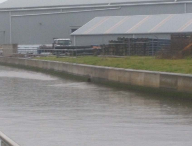
Figure E-67: Main plant outfall outlet on 18 June 2020
