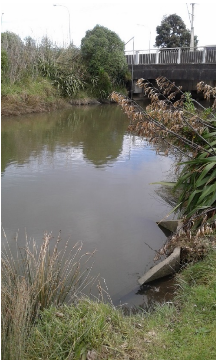
Figure E-11: Site C. Bell Road Bridge on 17 July 2019
