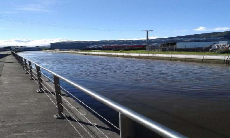
Figure E-1: Main plant overflow outlet on 15 July 2019
