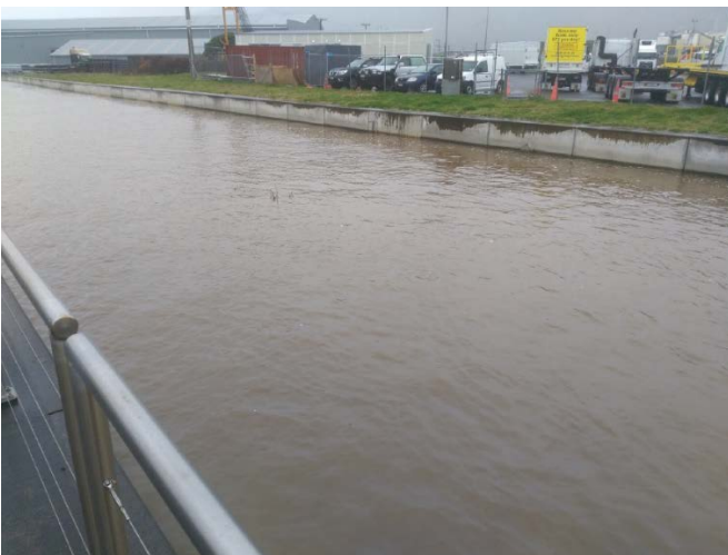
Figure E-60: Main plant overflow outlet on 05 June 2020
