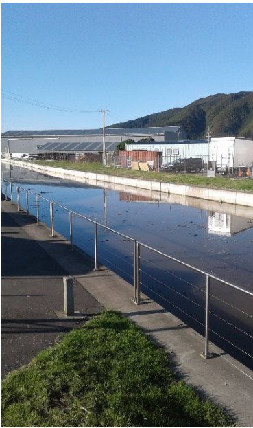
Figure E-54: Main plant overflow outlet on 06 May 2020
