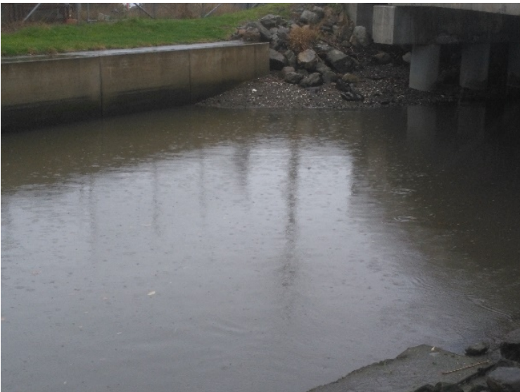
Figure E-68: Site A. Port Road on 18 June 2020
