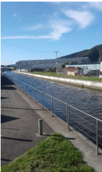
Figure E-57: Main pliant overflow outlet on 07 May 2020
