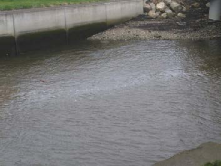
Figure E-74: Site A. Port Road on 20 June 2020
