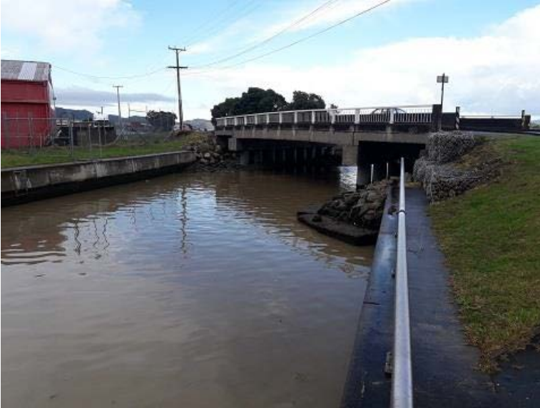
Figure E-6: Site A. Port Road on 16 July 2019
