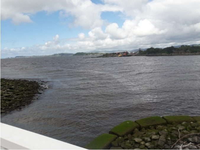
Figure E-29: Site A. Port Road on 12 November 2019
