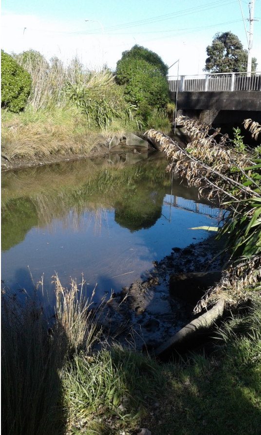
Figure E-4: Site C. Bell Road Bridge on 15 July 2019
