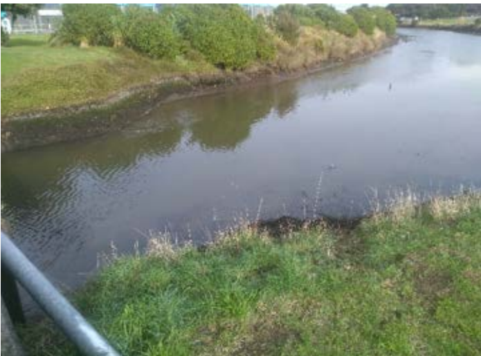
Figure E-66: Site C. Bell Road Bridge on 06 June 2020
