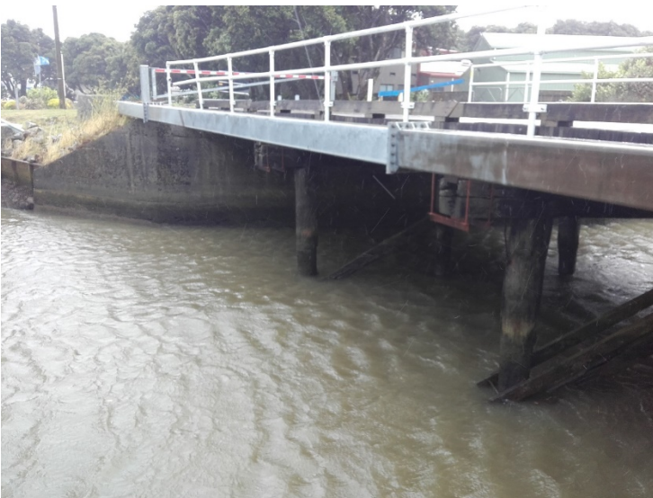
Figure E-46: Site C. Bell Road Bridge on 28 March 2020
