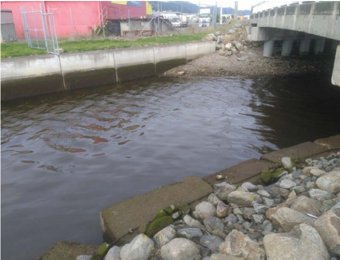
Figure E-64: Site A. Port Road on 06 June 2020
