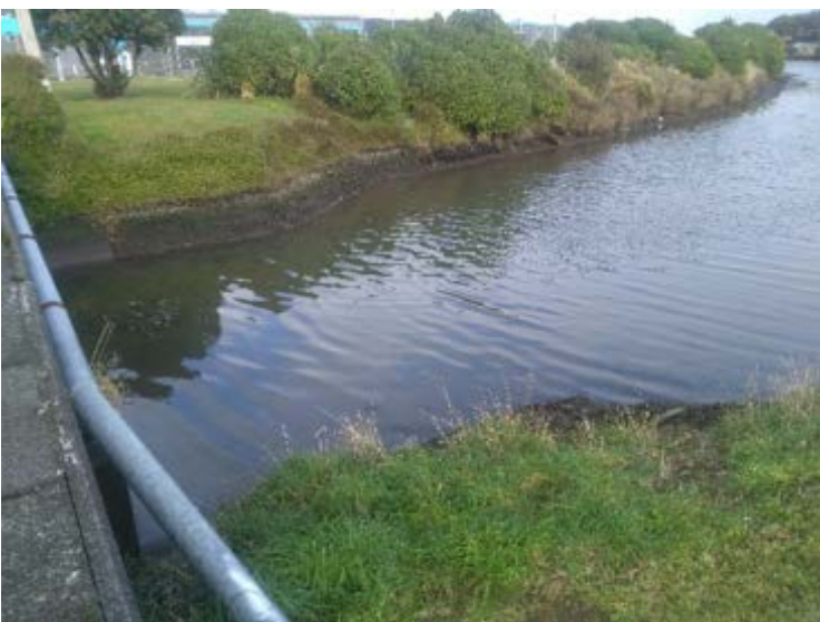
Figure E-76: Site C. Bell Road Bridge on 20 June 2020
