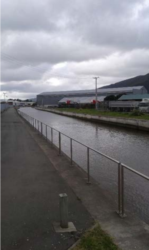
Figure E-16: Main plant overflow outlet on 14 August 2019
