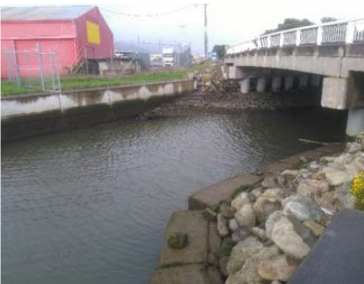
Figure E-80: Site A. Port Road on 21 June 2020
