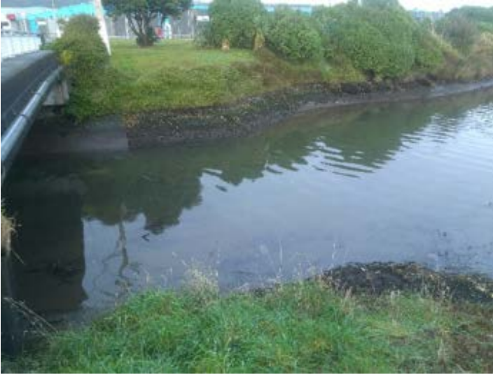
Figure E-79: Site C. Bell Road Bridge on 21 June 2020
