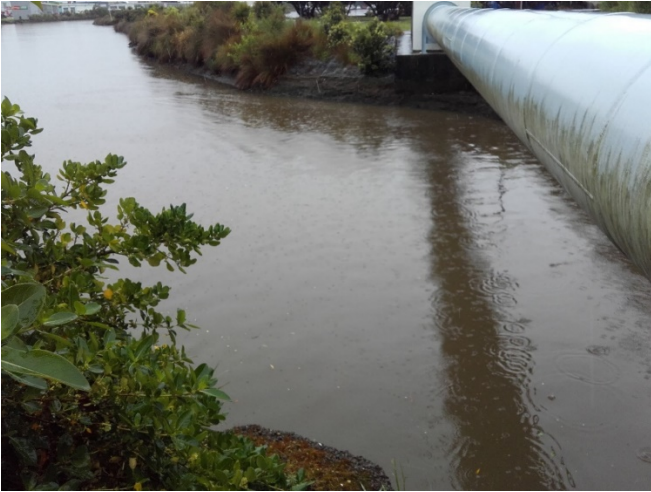
Figure E-27: Site C. Bell Road Bridge on 11 November 2019
