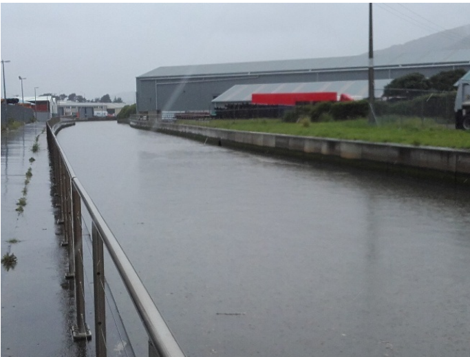
Figure E-24: Main plant overflow outlet on 11 November 2019
