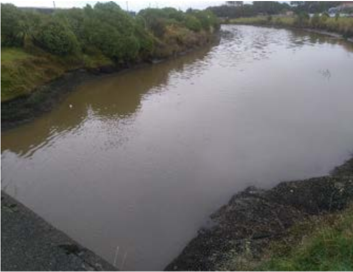
Figure E-72: Site C. Bell Road Bridge on 19 June 2020
