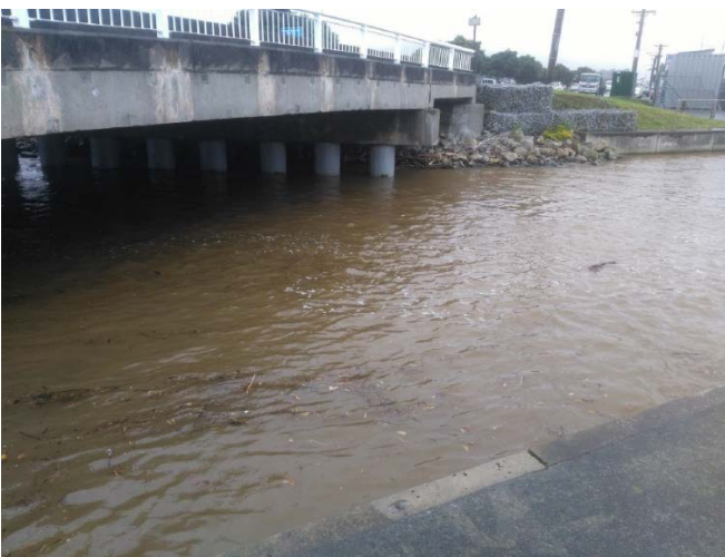
Figure E-61: Site A. Port Road on 05 June 2020
