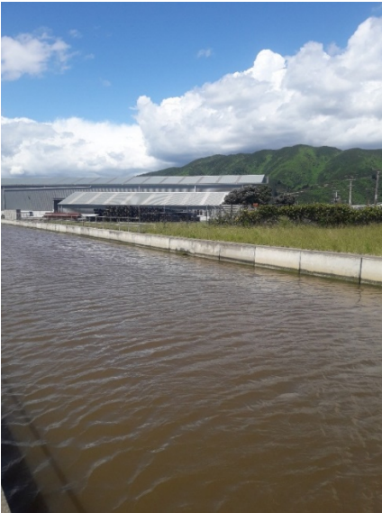
Figure E-36: Main plant overflow outlet on 09 December 2019
