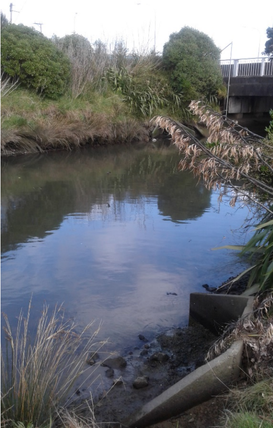
Figure E-19: Site C. Bell Road Bridge on 14 August 2019
