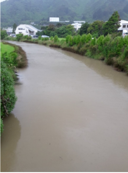
Figure E-35: Site C. Bell Road Bridge on 08 December 2019
