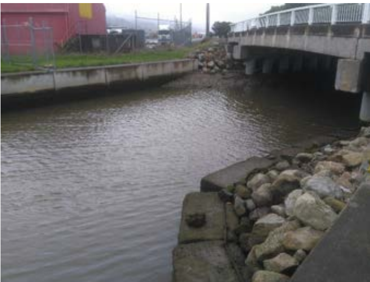
Figure E-70: Site A. Port Road on 19 June 2020
