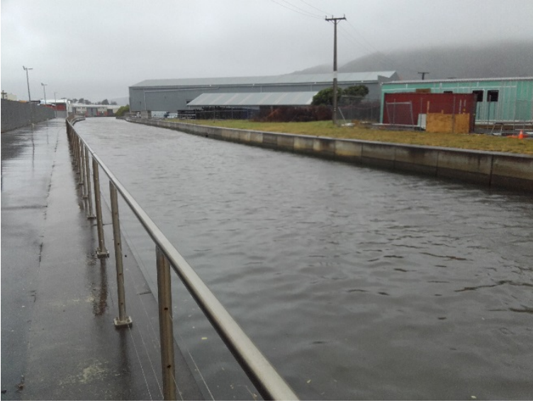
Figure E-47: Main plant overflow outlet on 29 March 2020
