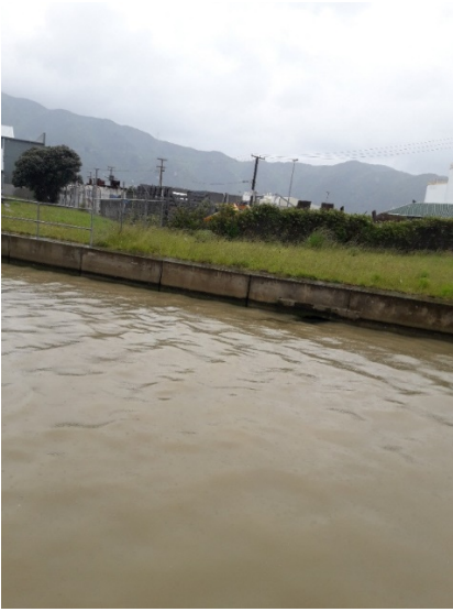
Figure E-32: Main plant overflow outlet on 08 December 2019
