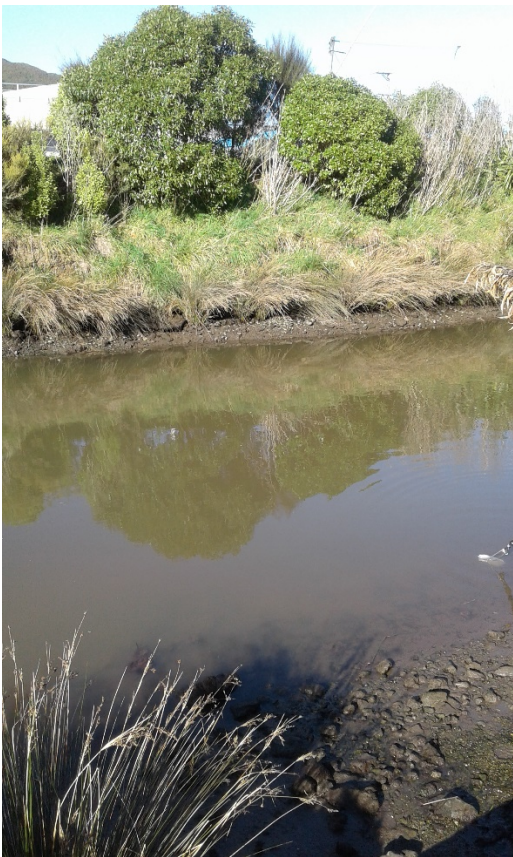
Figure E-15: Site C. Bell Road Bridge on 13 August 2019
