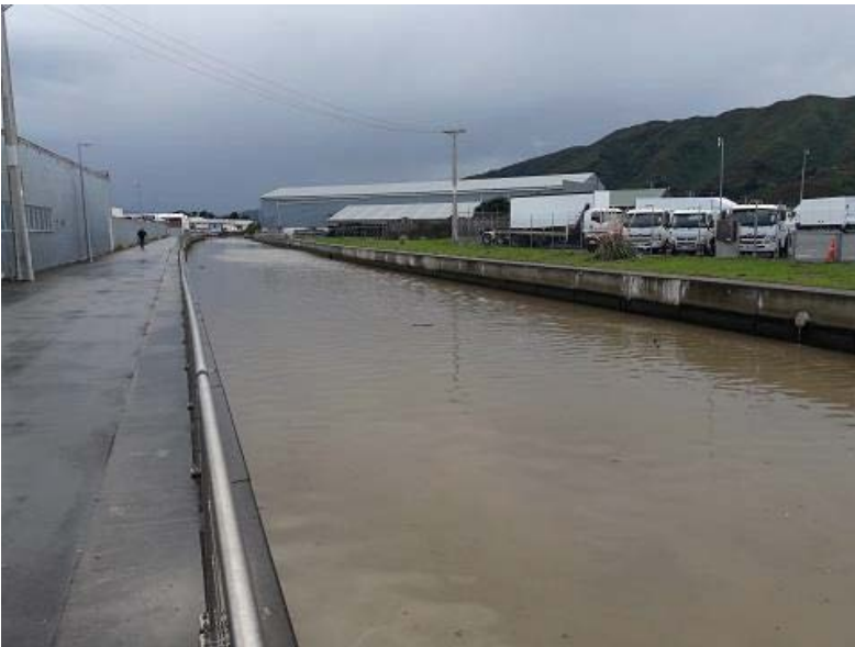
Figure E-5: Main plant overflow outlet on 16 July 2019
