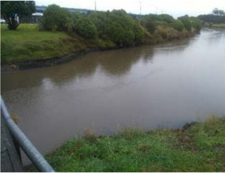
Figure E-70: Site C. Bell Road Bridge on 18 June 2020
