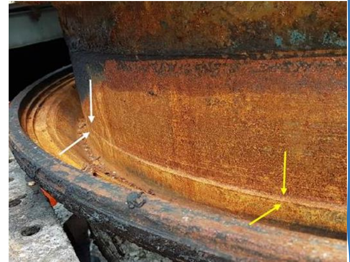
The image above shows where the bearing track inside a clarifier at Moa Point has worn away. Below, new blowers installed at the Porirua treatment plant, to provide oxygen for effective treatment processes. Replacing key assets before they fail is a key outcome of proactive asset condition assessment
