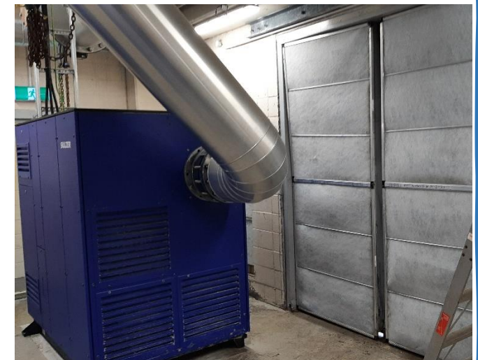
The image above shows where the bearing track inside a clarifier at Moa Point has worn away. Below, new blowers installed at the Porirua treatment plant, to provide oxygen for effective treatment processes. Replacing key assets before they fail is a key outcome of proactive asset condition assessment
