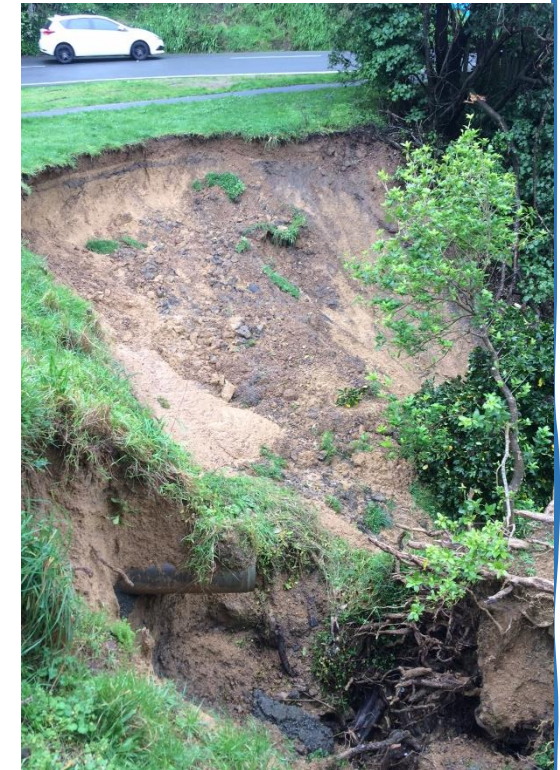
Bursts and leaks are reactive events that can have a significant impact on operational budgets
