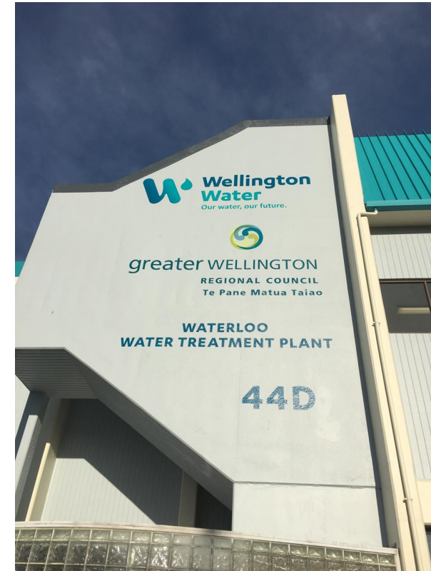
Waterloo treatment plant
