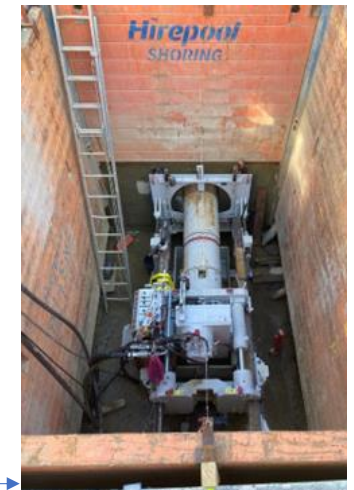
The drilling machine in use, approx. 5m underground on Taranaki Street.
