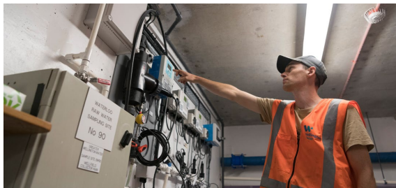
Operator monitoring the raw water sampling at the Waterloo Water Treatment Plant
