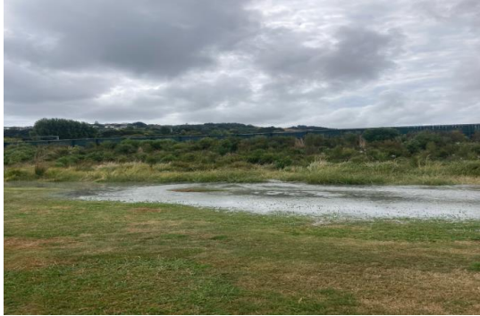
Site of the burst drinking water pipe which feeds into the Plimmerton Reservoir
