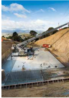
Construction of a new reservoir at Mt Albert Park, Wellington
