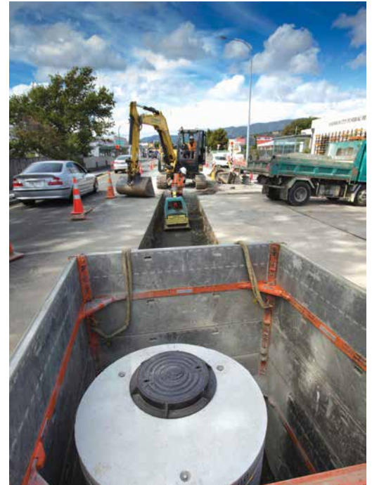
Upgrading a wastewater pipeline in Fergusson Drive, Upper Hutt
