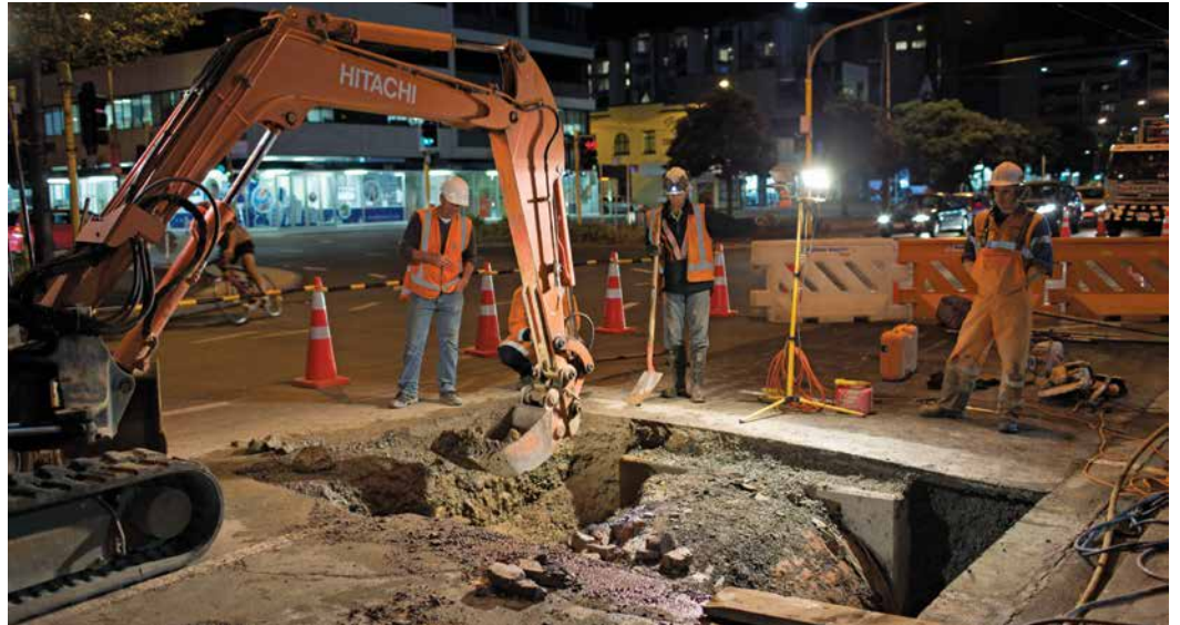
Repairing and strengthening an aging stormwater main in Kent Terrace, Wellington
