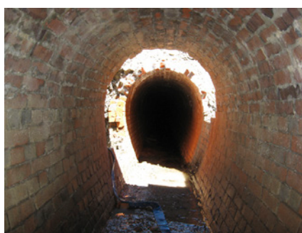
Te Aro culvert – Ovoid shape brick culvert constructed in the 1930s
