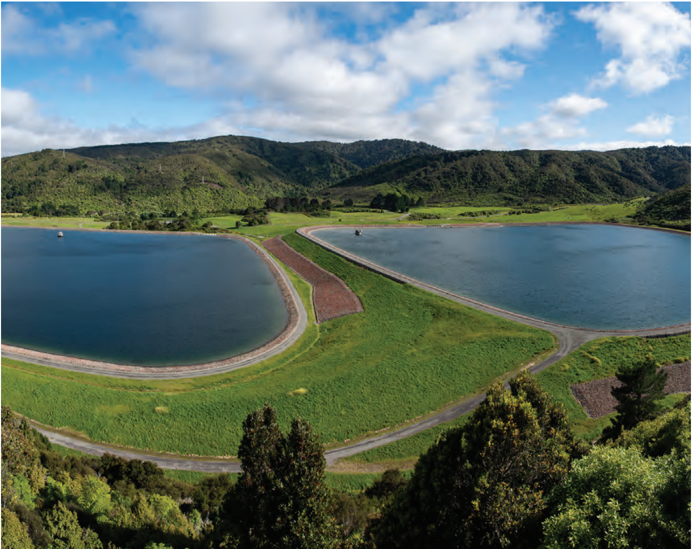
The storage water in our Stuart Macaskill Lakes is used to supplement supply when we can't take enough water from the rivers or aquifer to meet demand.
