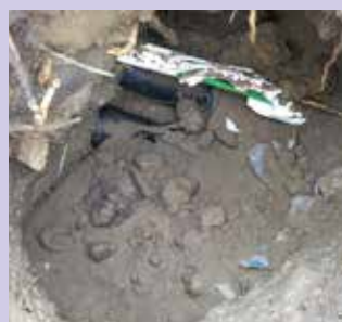
[Left] Having services buried right next to, on top or underneath each other increases the risk of damage. [Right] Citycare staff joined us on the ground to let people know and deliver safe water.
