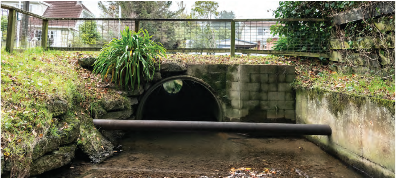
Sunbrae Drive Culvert will be twice the size it is now.
