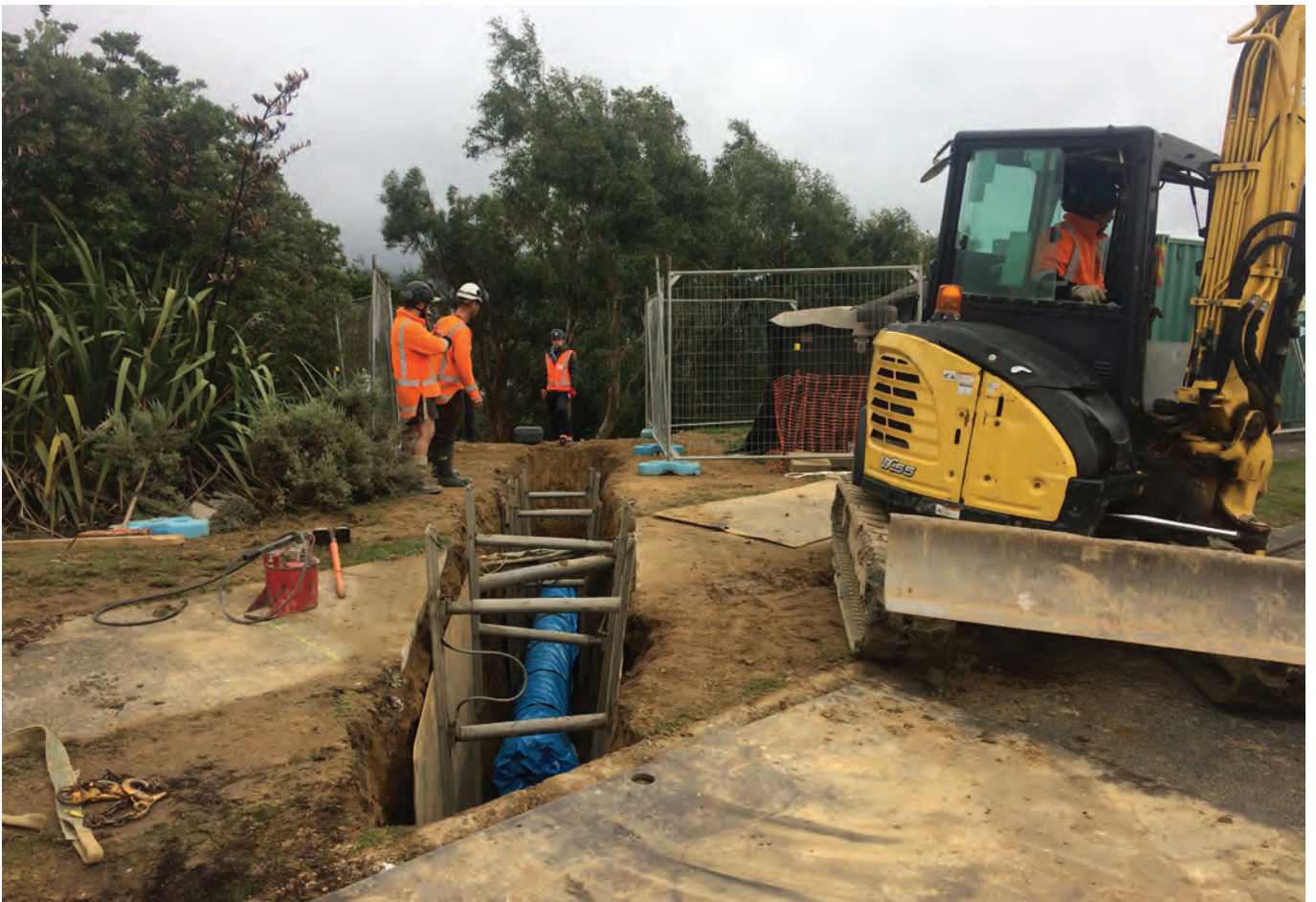
Kurimoto Ltd manufacture an earthquake resilient pipe, which allows the type of joint movement which can absorb severe shocks. It is incredibly important for us to develop high quality resilient options for our region's pipelines. We are currently using this pipe in a trial project, the Porirua Branch Extension, which will be completed between April and early August.
