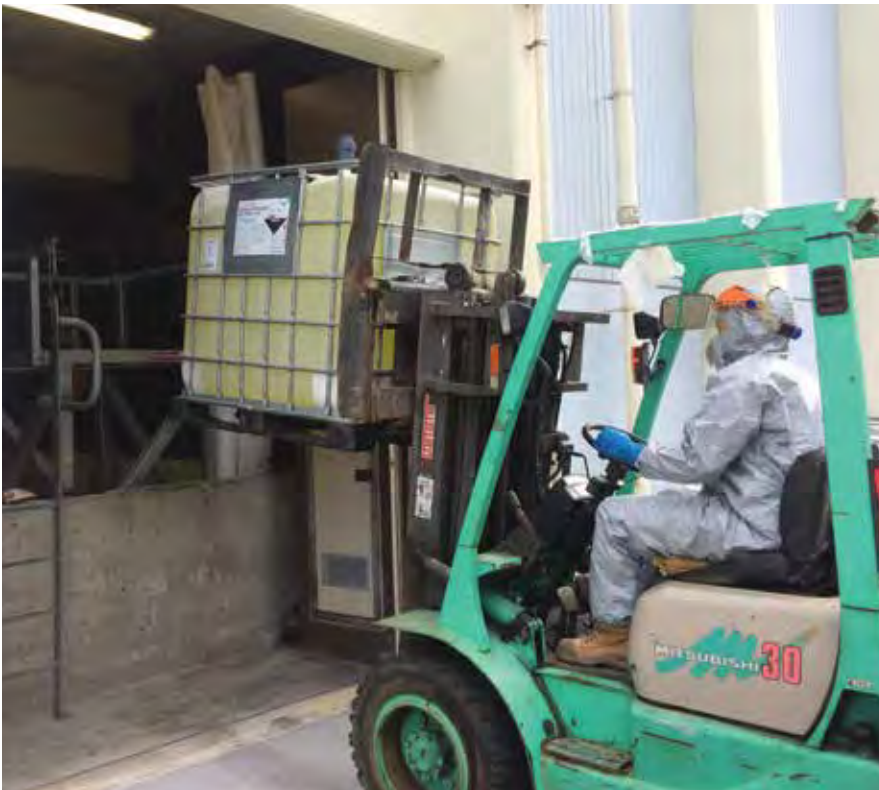
Loading a container of sodium hypochlorite (liquid chlorine used for water supply disinfection) into Waterloo Drinking Water Treatment Plant's chlorination room.
