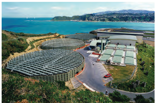
Moa Point Wastewater Treatment Plant.
