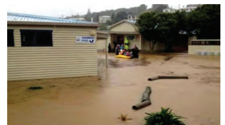
A flooding event in May 2016, caused an evacuation (by rubber dinghies!) of the school and damage to school buildings.
