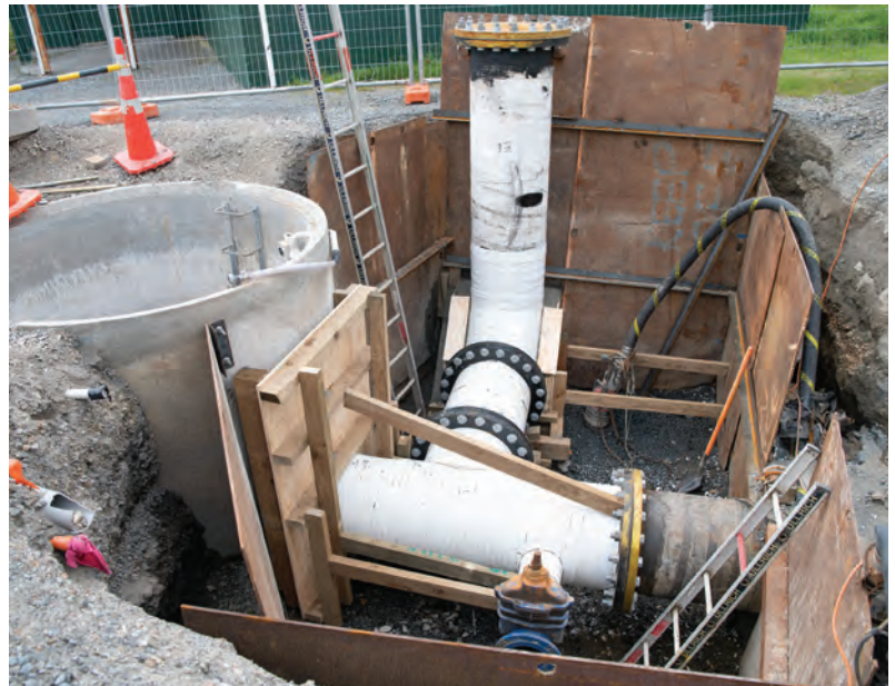
Installation of ultraviolet treatment at our Gear Island Water Treatment Plant.
