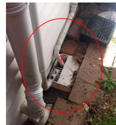
Mis-connections into the wastewater network increase the volume of water in the system, and the risk of overflows.
