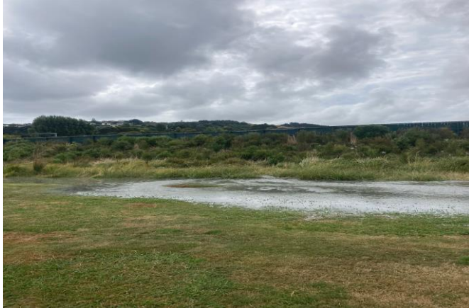
Site of the burst drinking water pipe which feeds into the Plimmerton Reservoir
