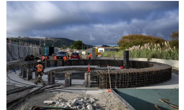
Sections of the new wastewater storage tank in Porirua being built. Once completed the tank will hold wastewater during times of heavy rain to reduce overflows into the environment.
