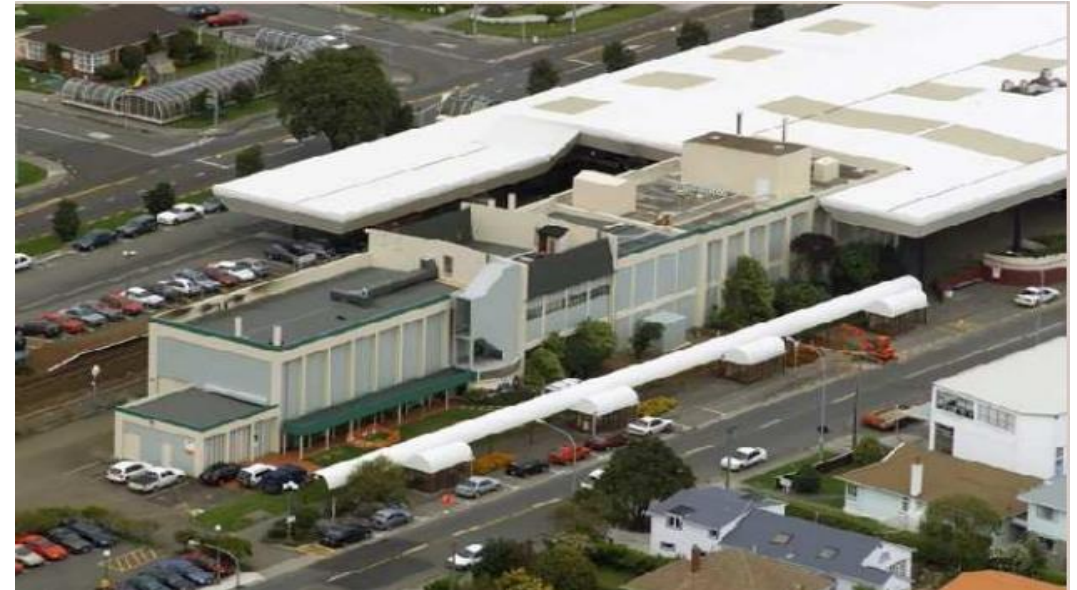
The Waterloo Water Treatment Plant, which supplies around 40% of the Wellington metropolitan region's water supply.
