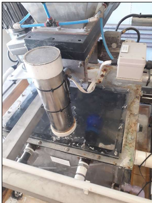
Figure 4 Te Marua WTP: Powder Feeder and Mixing Tank
