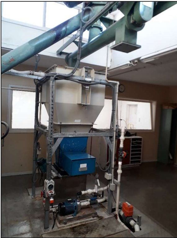
Figure 15 Wainuiomata WTP: SSF Powder Day Hopper
