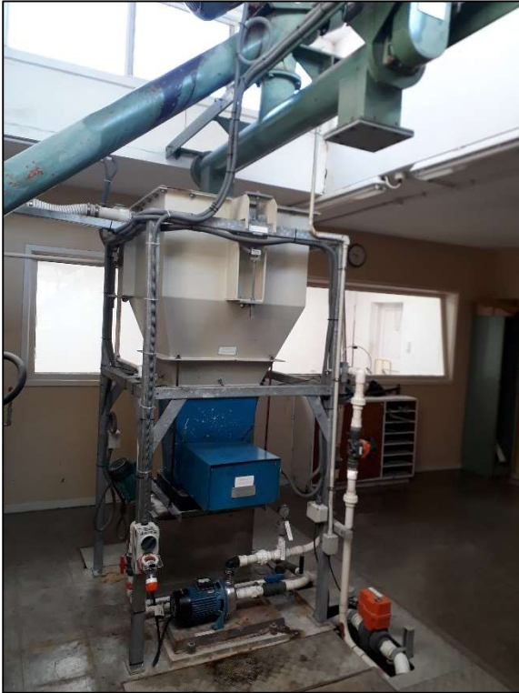
Figure 15 Wainuiomata WTP: SSF Powder Day Hopper
