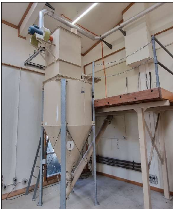
Figure 2 Te Marua WTP: SSF Powder Storage Hopper (note ladder and lack of handrail on platform)
