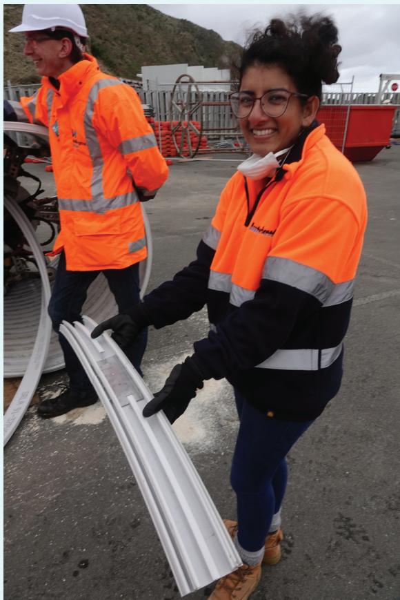
A durable, long-term solution: Project Manager Saadia Ali with a section of the PVC used to line the interceptor.
