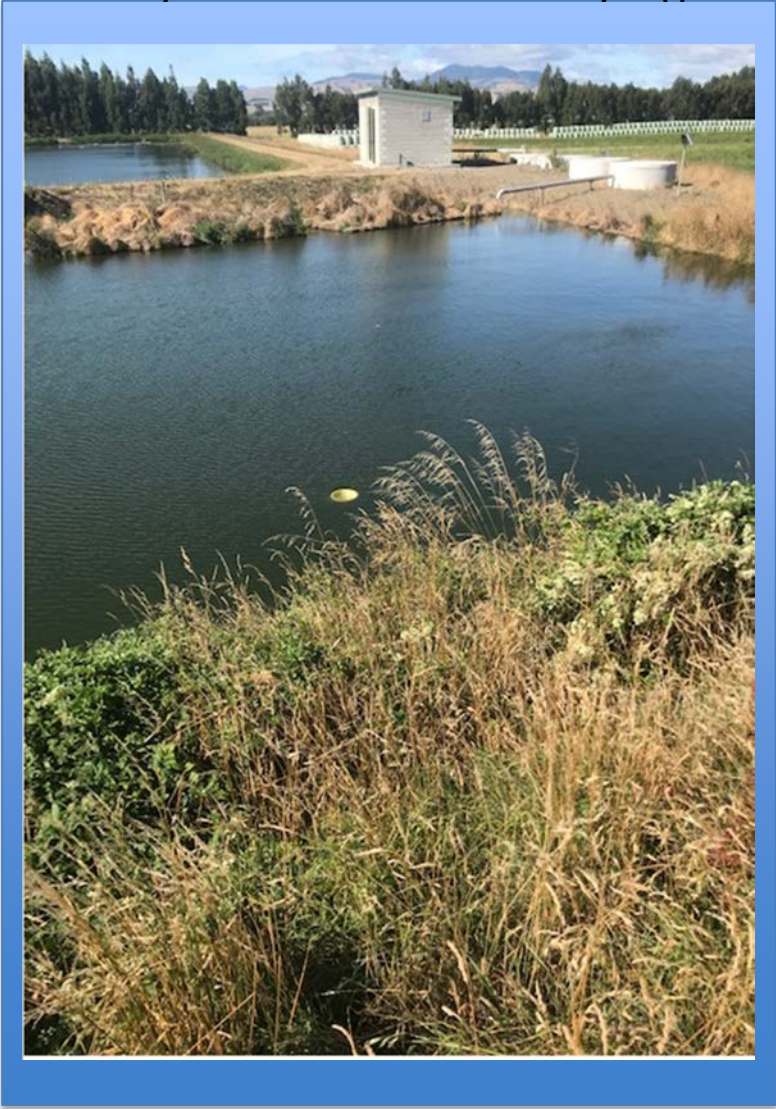
January 27 11:30 – Overflow had already stopped
