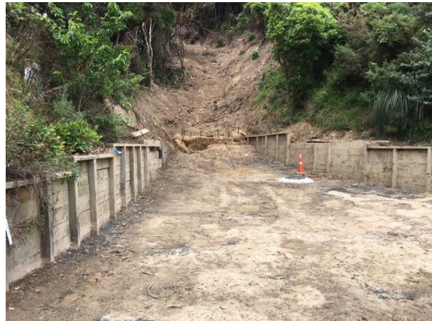
Hundreds of tonnes of earth needed excavation in Leeward Drive, Porirua
