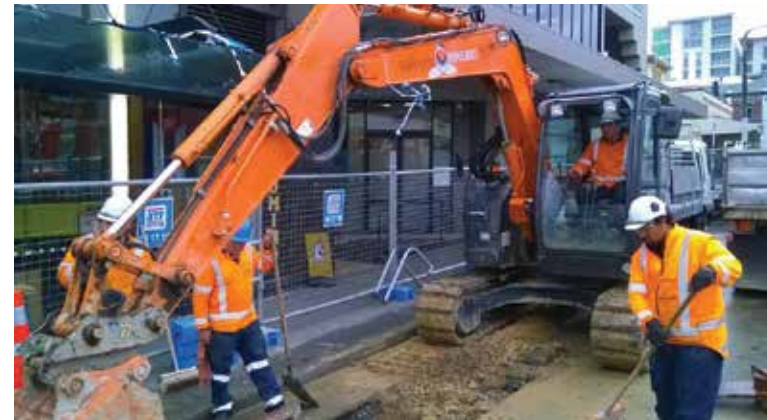
Work underway in Cuba Street.
