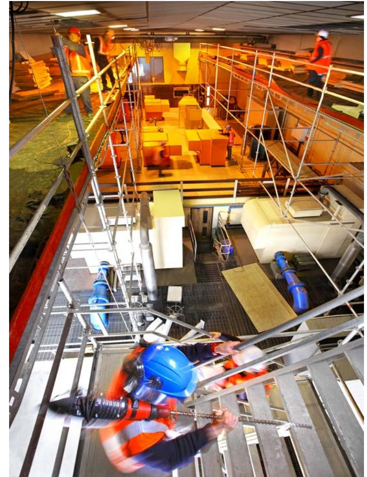
Structural strengthening of the Waterloo treatment plant's motor hall
