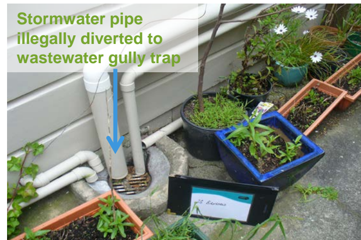
Private stormwater downpipes diverted to wastewater gully traps are a major cause of increased wastewater network loading, and possible overflows, during wet weather.
