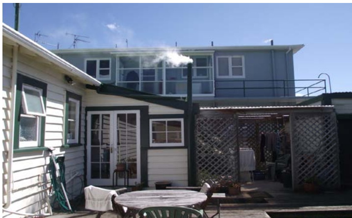
Smoke pumped into a stormwater main leaves a wastewater ventilation pipe -- evidence of a cross-connection that will be affecting receiving water quality.
