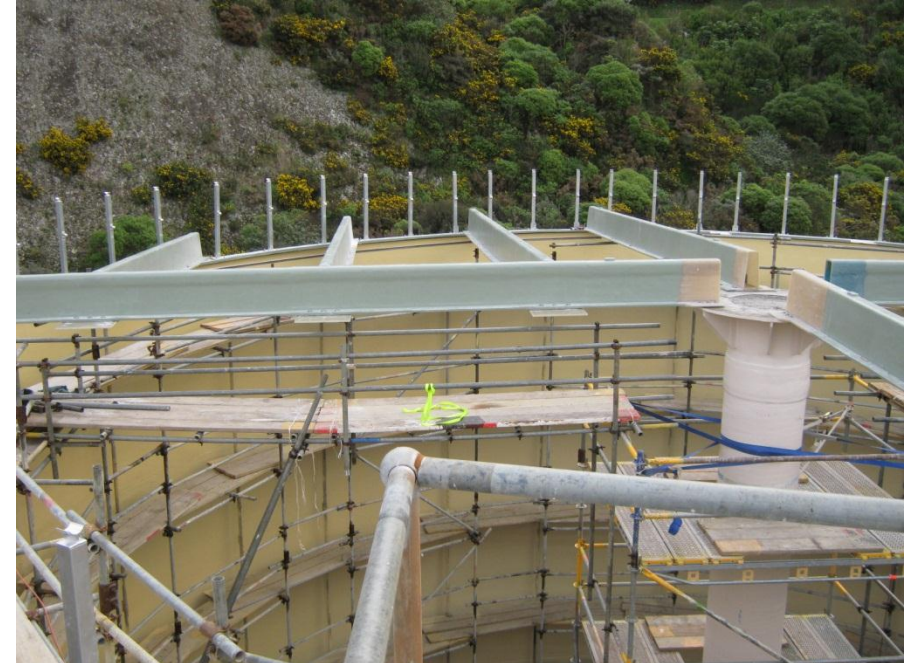
Sludge holding tanks at Carey's Gully were relined and re-roofed recently.
