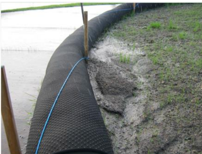
Photo 1 Silt or Filter Socks used as edge protection (example 1)
