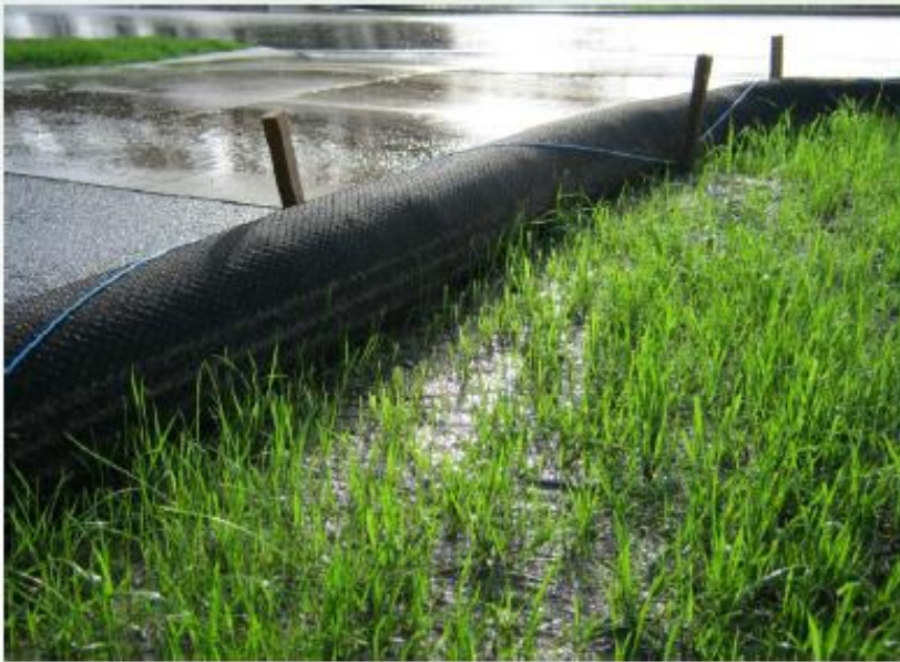
Photo 2 Silt or Filter Socks used as edge protection (example 2)
