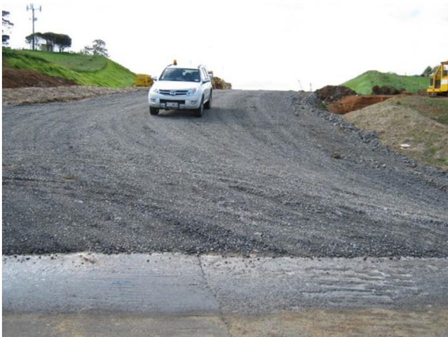
Photo 4 Typical appearance of a stabilised entranceway
