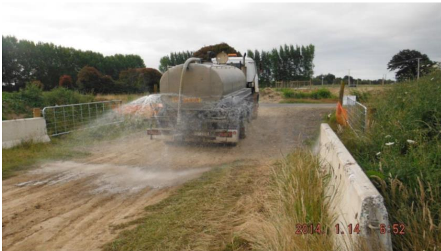
Photo 8 Water Cart in operation
