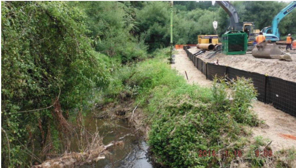
Photo 5 Super Silt Fence
