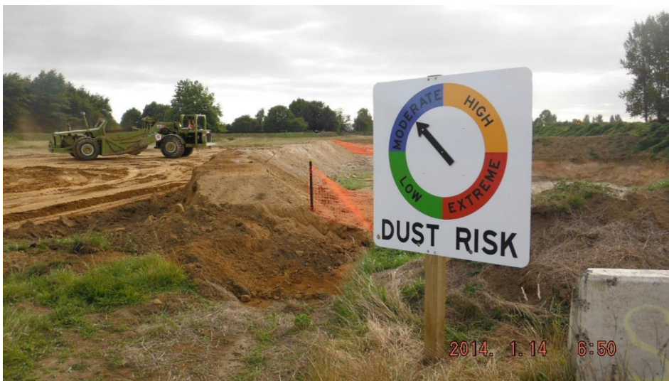
Photo 9 Dust risk signs will assist with communicating the risk to construction staff
