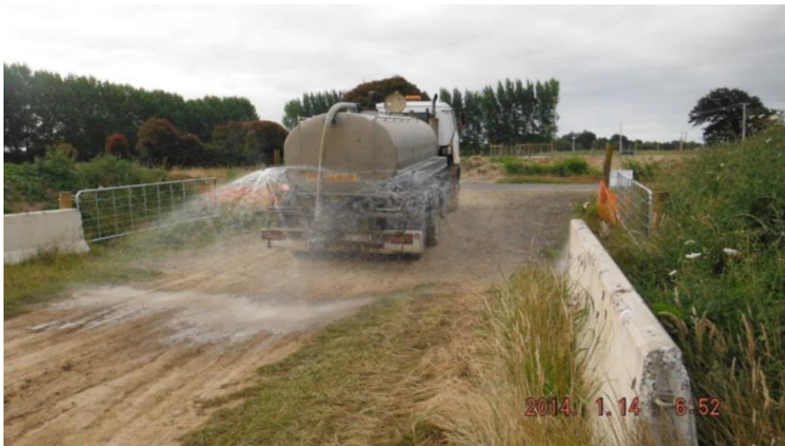
Photo 8 Water Cart in operation
