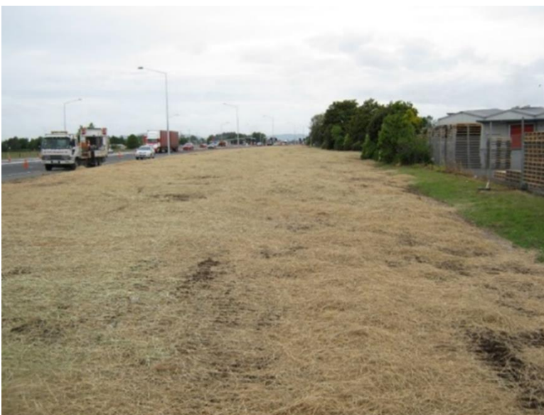
Photo 3 Hay Mulch applied to large surfaces following completion to stabilise.
