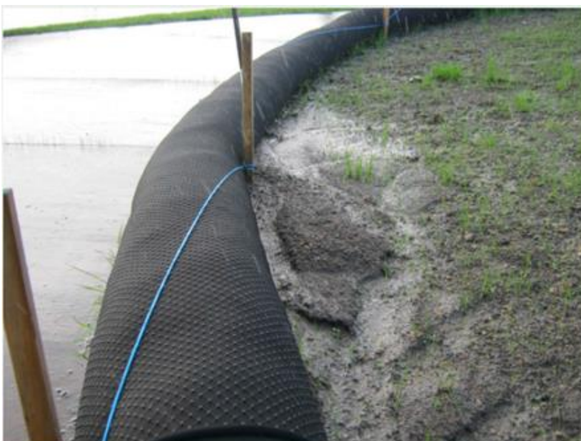
Photo 1 Silt or Filter Socks used as edge protection (example 1)
