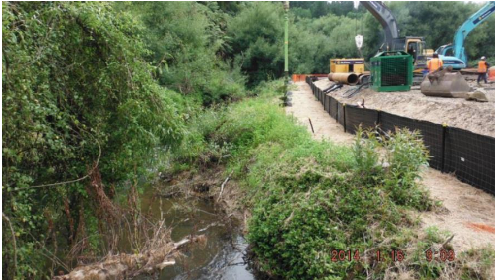
Photo 5 Super Silt Fence
