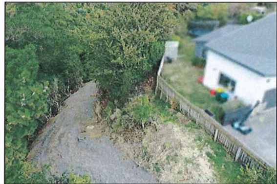
Figure 2: Drone image showing cut proximity to No. 23. Note existing vegetated slope already in place.
