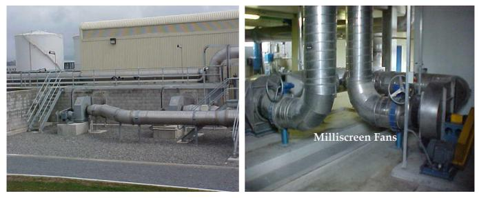
The millsicreen fans are New York Blower (NYB) 188 class 111. The operating point for each fan is around 1.8m3/s at 2000Pa. Refer photo above and close up below.
