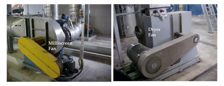
The dryer fan is an Aerotech MVM 270 driven by a 30 kW variable speed motor. The design operating point is around  $3.5 \text{ m}^3/\text{s}$  at 300 Pa. Refer Photo above.
