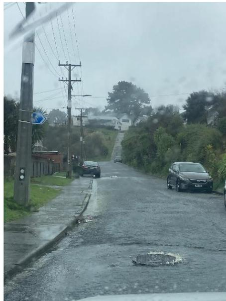
Figure 2: Uncontrolled overflow observed on 19<sup>th</sup> August 2022.
