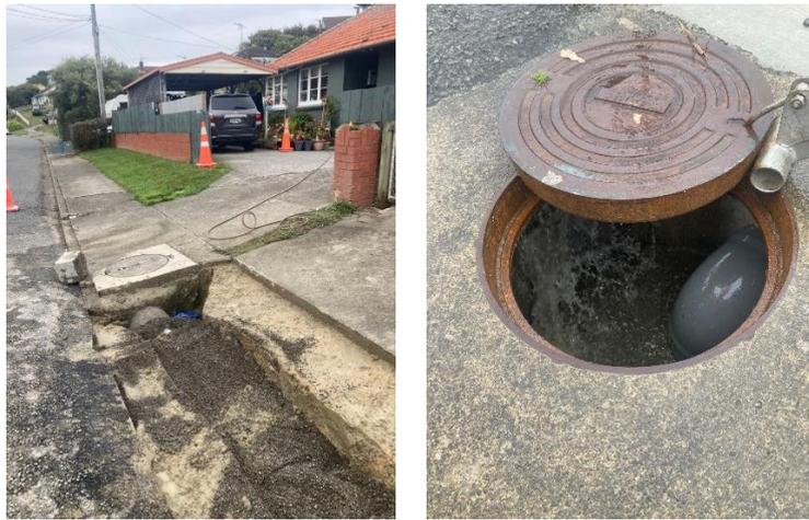
Figure 1 Constructed overflow installed in Thompson Grove
