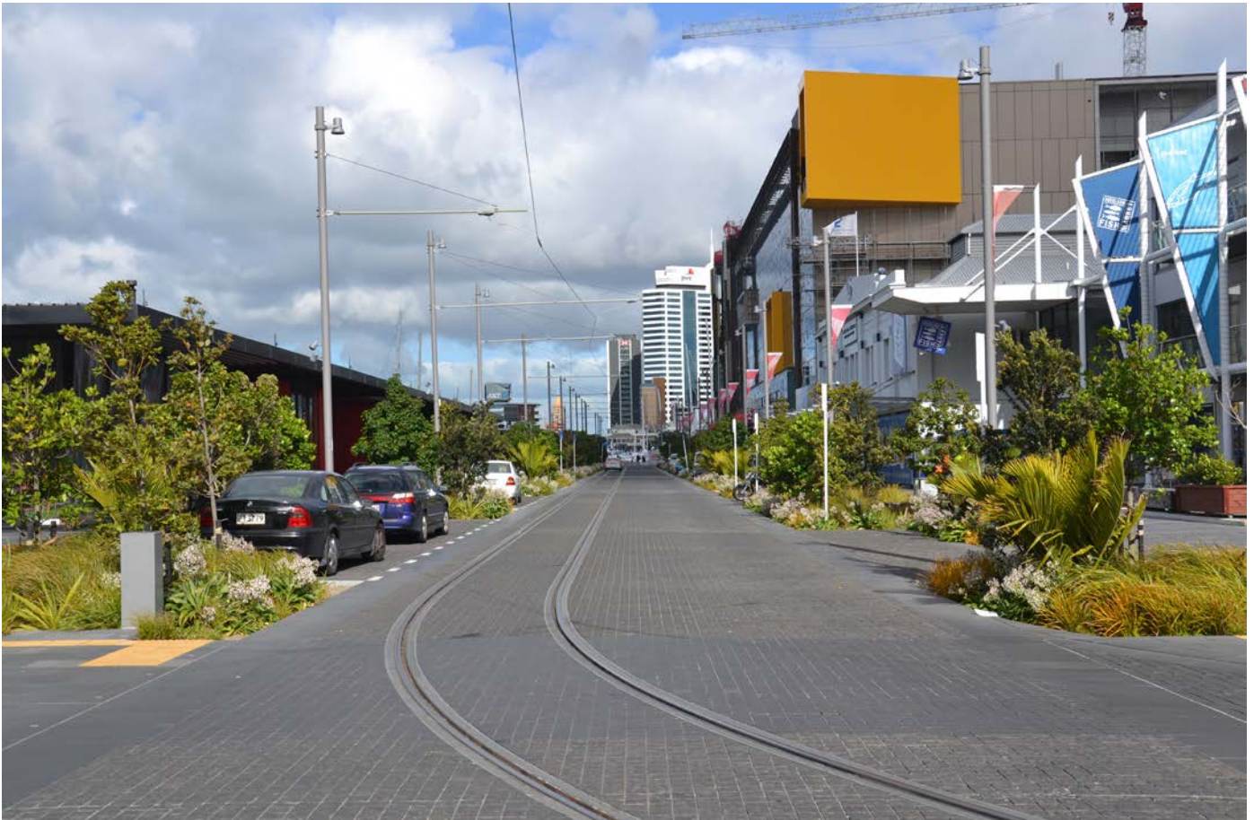
Figure 27: Example of Bioretention in pedestrian areas. Wynyard Quarter, Auckland.
