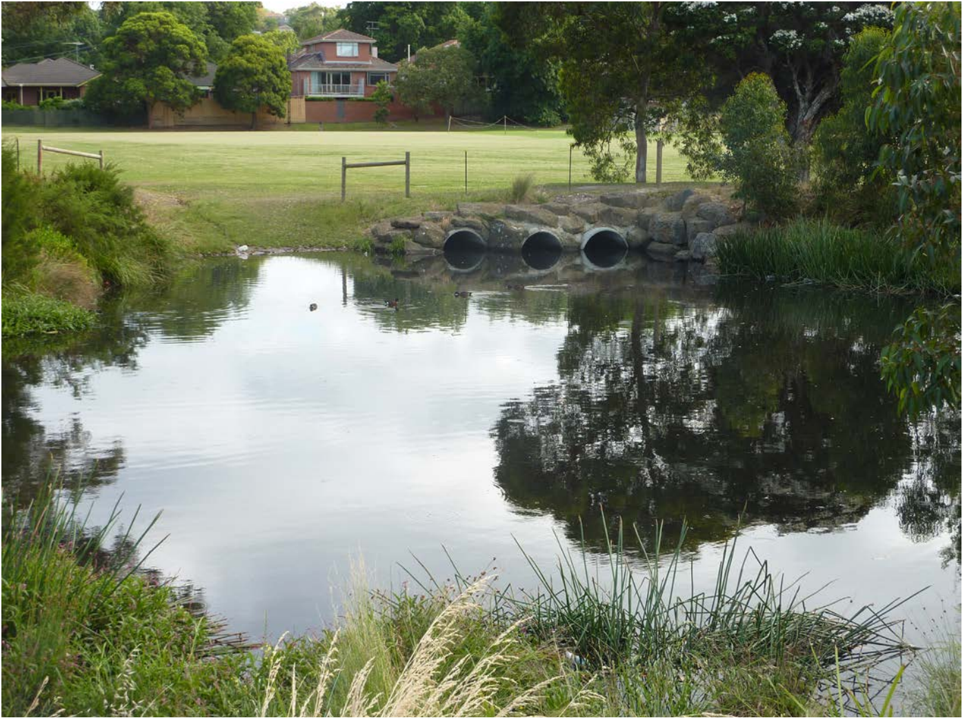
Figure 15: Wetland forebay with maintenance access left of inlet pipes.
