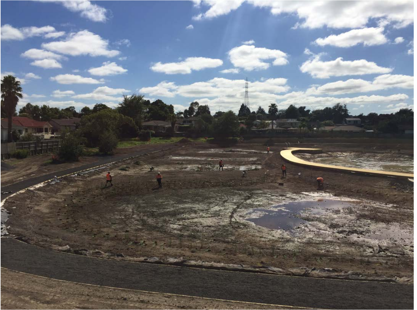
Figure 23: Planting into substrate (topsoil stripped from site and laid over GCL liner).
