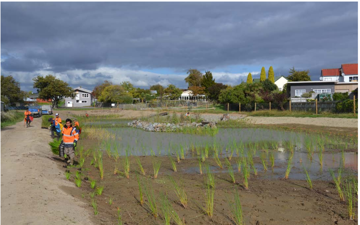
Figure 25: Planting of completed wetland with water level lowered.
