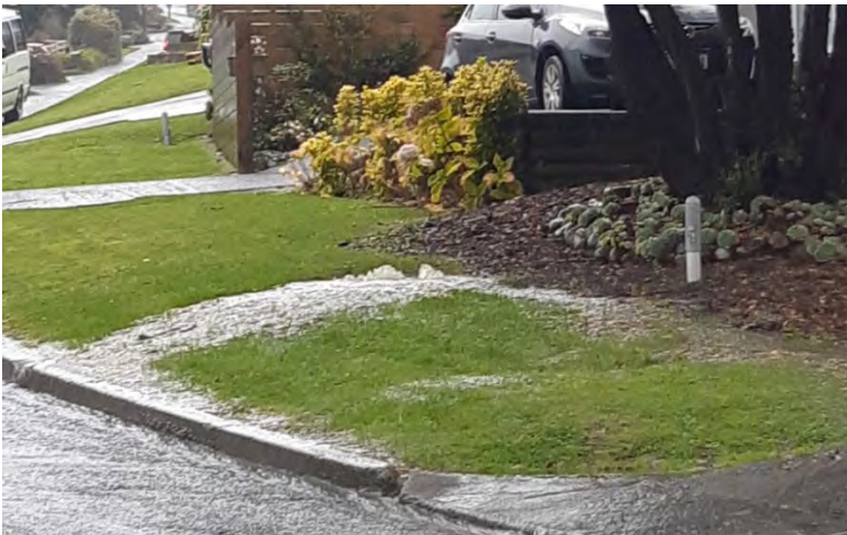
Figure 2-5: View of an uncontrolled overflow from a manhole into a nearby kerb and channel
