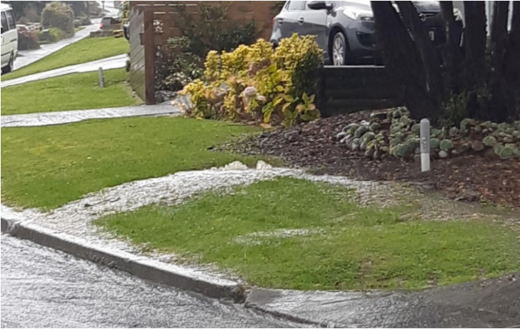
Figure 2-1: View of an uncontrolled overflow from a manhole into a nearby kerb and channel
