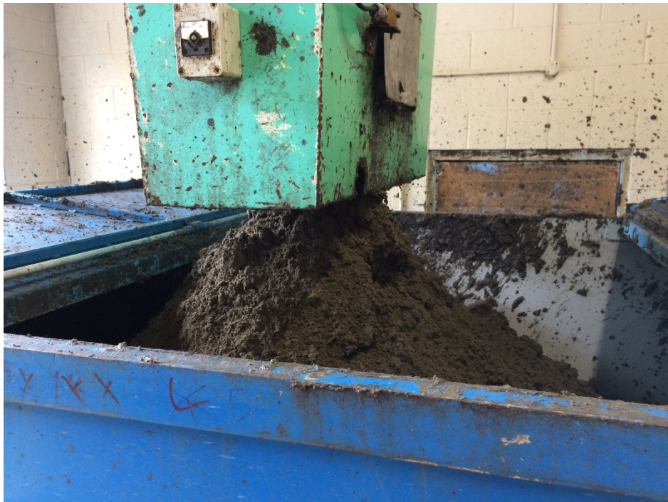
Figure 10: Dewatered sludge awaiting covering and transport for landfill disposal
