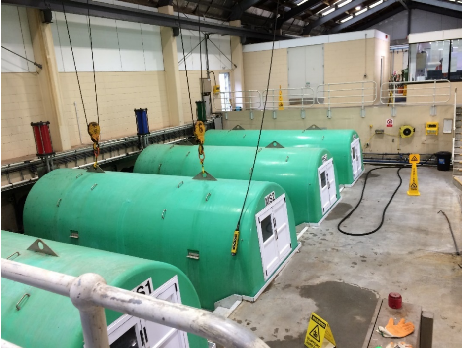
Figure 8: The Milliscreening Hall, with fibreglass covers over the screens to minimise H 2 S/ odour release
