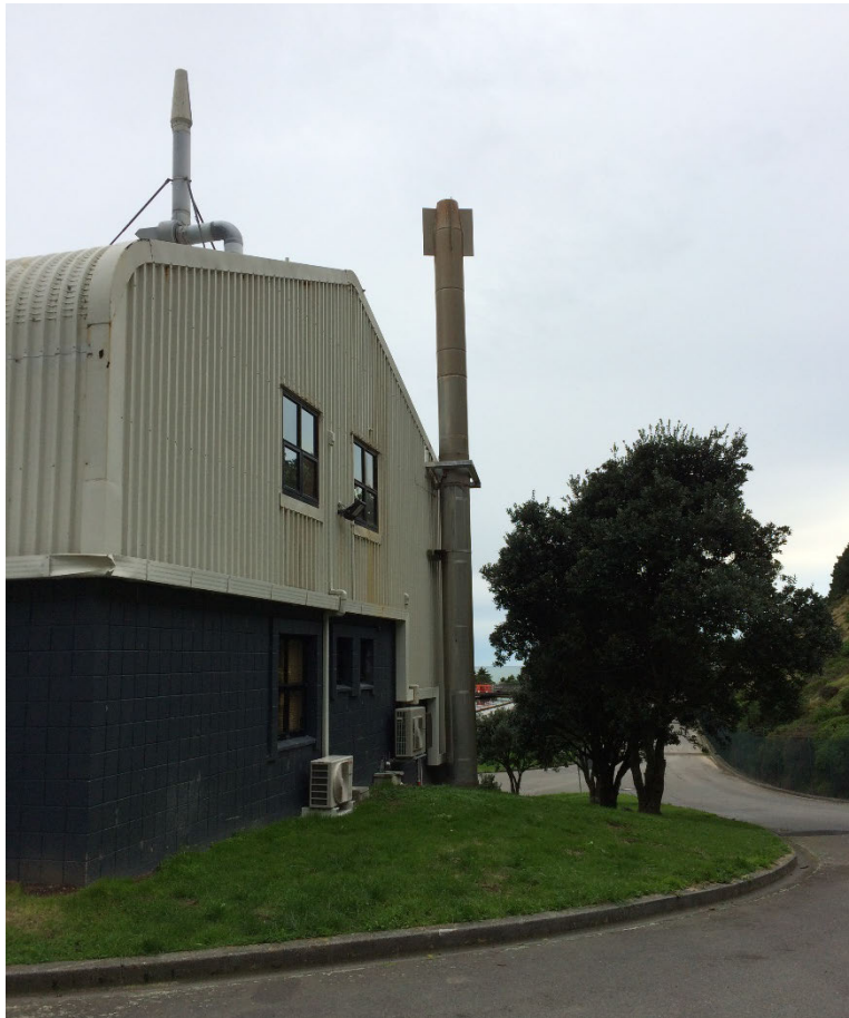
Figure 7: North-east corner of WWTP building showing the 10m discharge stack
