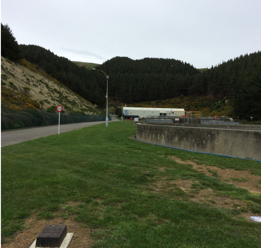
Figure 6: General View of the Porirua WWTP looking to the south east along the access road
