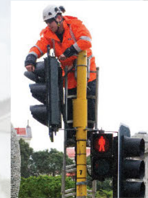
Correct Steps facing the work activity
