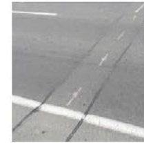
Reinstated asphalt
